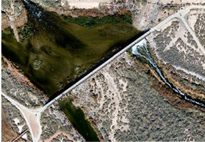
Photo 1 - 810F (2008) Upper Diversion Weir
