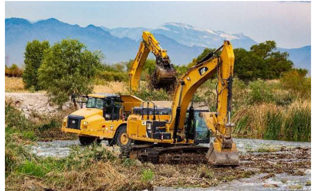
Weir maintenance work on Las Vegas Wash
